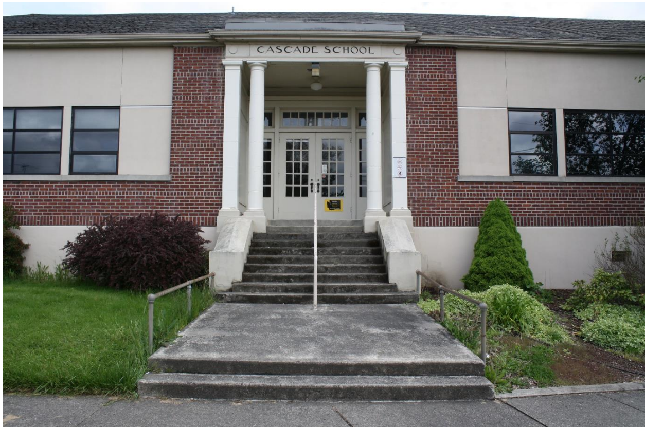
Figure 2 North Elevation Entry, View South
