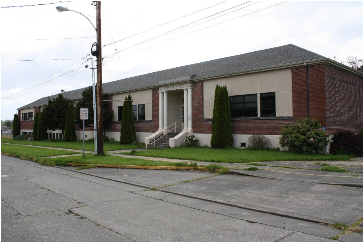
Figure 3 South Elevation, View Northwest
