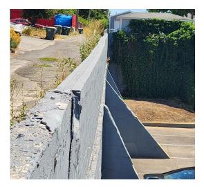
The parking lot retaining wall has also experienced persistent water seepage through the wall. Due to the ongoing water, it has cracked in several places, and it has shifted, causing it to lean towards the parking lot. The paint continues to peel off in the areas where the water seeps
