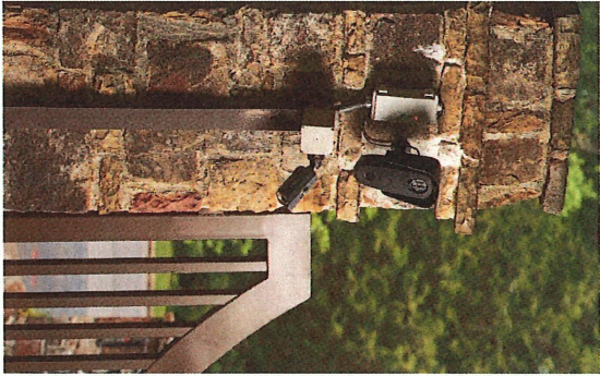
Electric & Existing Structure / Pole
