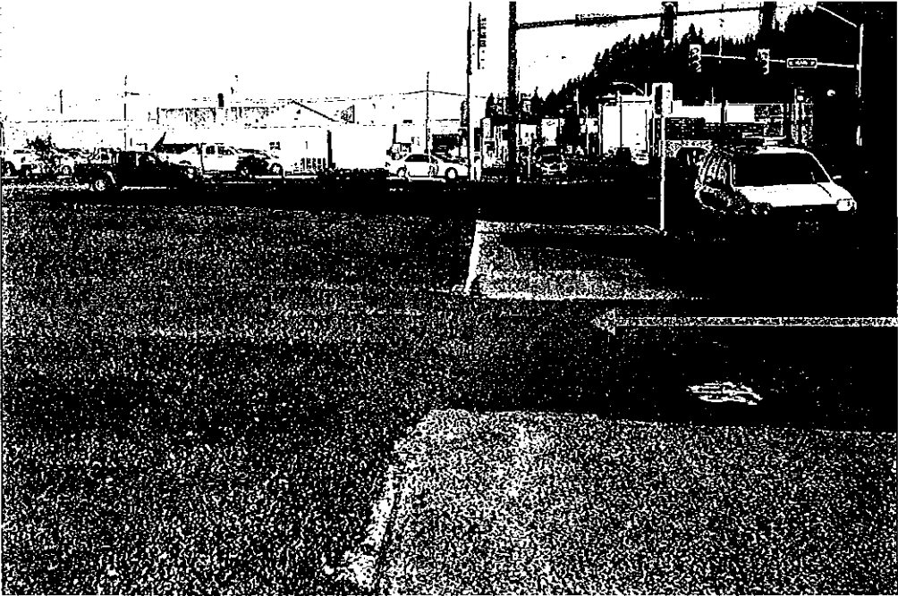
Alleyway from SW Chehalis Ave. looking northward
