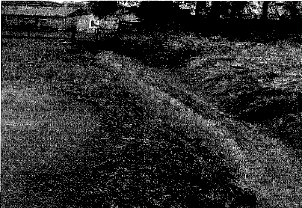
Storm Water runoff going towards residential neighborhood
