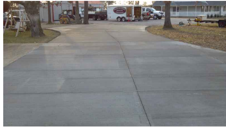
6 BROOM FINISH PCC SIDEWALK N.T.S.
