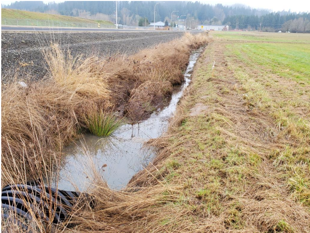
Existing ditch parallel with Rush Road, facing north.
