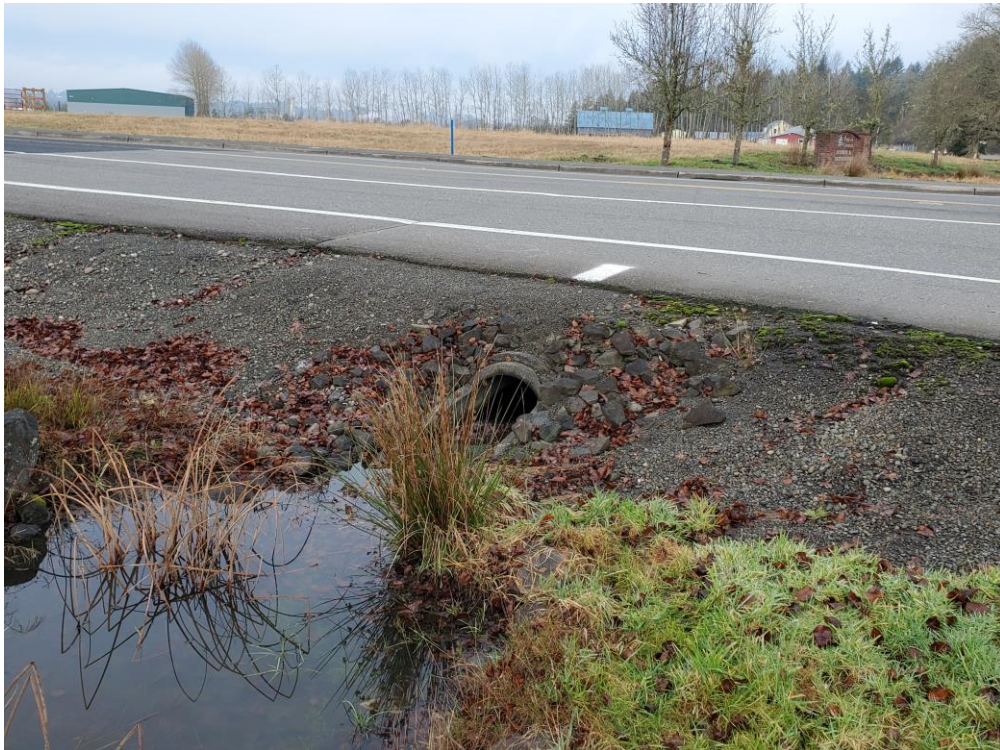
Concrete culvert near intersection of Rush Road and Jackson Highway.
