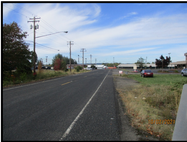
Photograph 4: Looking west on Exhibitor Road from the bridge over Salzer Creek. Southern site access on right.
