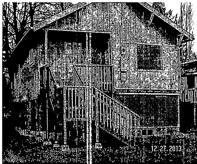
FRONT - SOUTH VIEW
