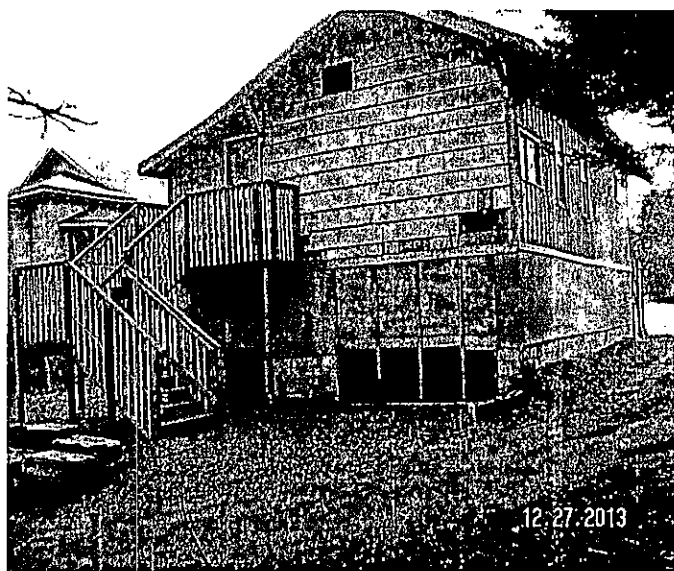
REAR - NORTH VIEW
