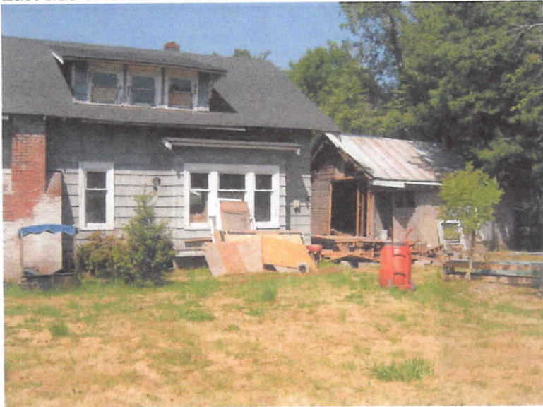
East side of House 7-24-08
