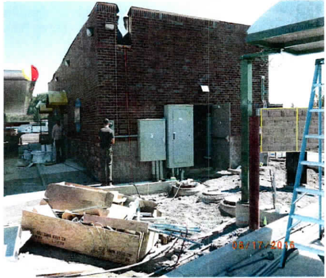
RIGHT VIEW – LOOKING SOUTHEAST
