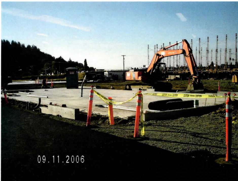
QUIZNOS, COLDSTONE 1640, 1644, AND 1648 NW LOUISIANA FROM NORTHWEST
