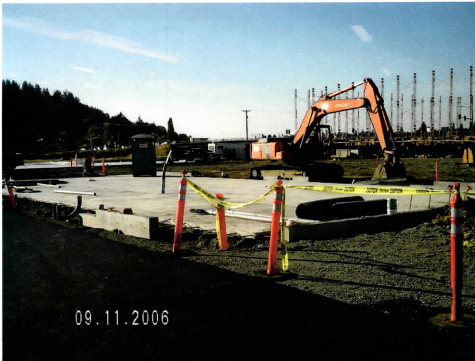
QUIZNOS, COLDSTONE 1640, 1644, AND 1648 NW LOUISIANA FROM NORTHWEST
