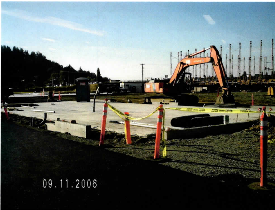
QUIZNOS, COLDSTONE 1640, 1644, AND 1648 NW LOUISIANA FROM NORTHWEST
