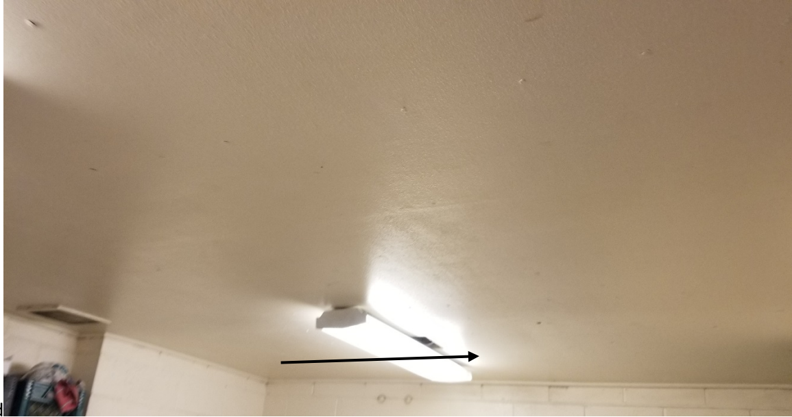
Typical ACM skim coat on GWB ceiling. Rm's 102 – 105, 112, 114 – 119, 120, & 122 – 126
