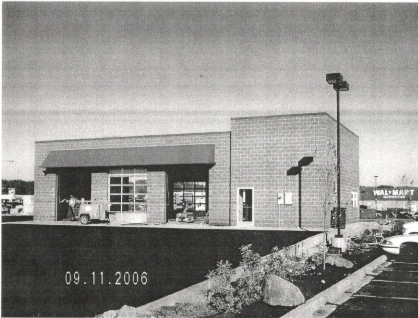
JIFFY LUBE FROM NORTHEAST
