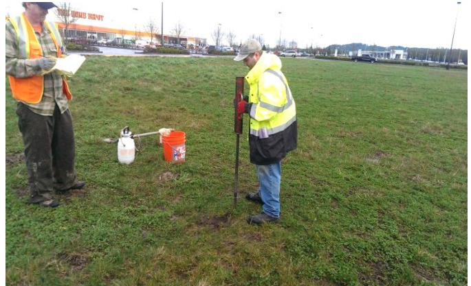
Photo 5. DCP Testing at DCP location P-1
