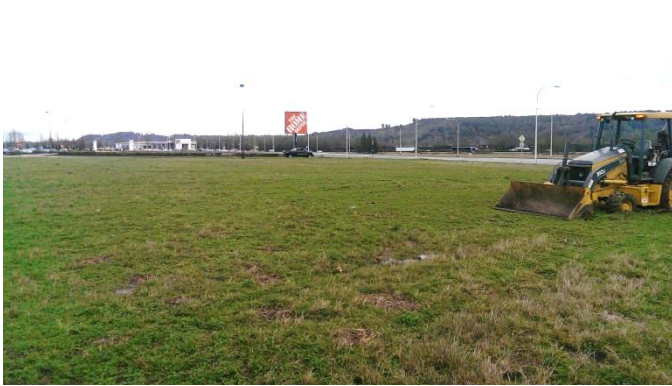
Photo 1. Looking East near West Corner of site
