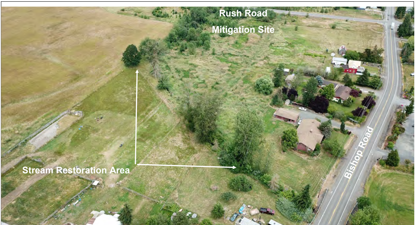
Above: Aerial view east, June 2018.
