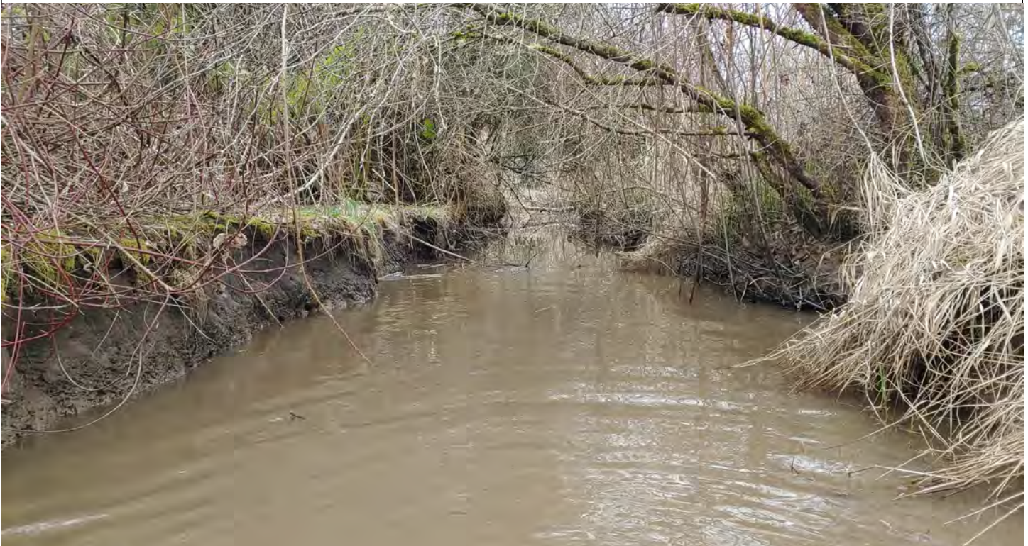
Below: (Photopoint 9) View east showing incised stream channel, March 2019
