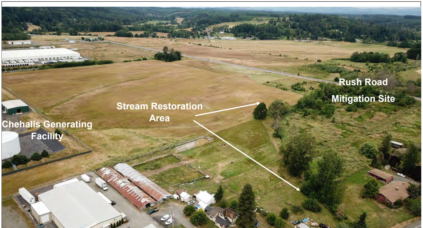
Above: Overview of Berwick Creek restoration project. Aerial view northeast June 2018.
