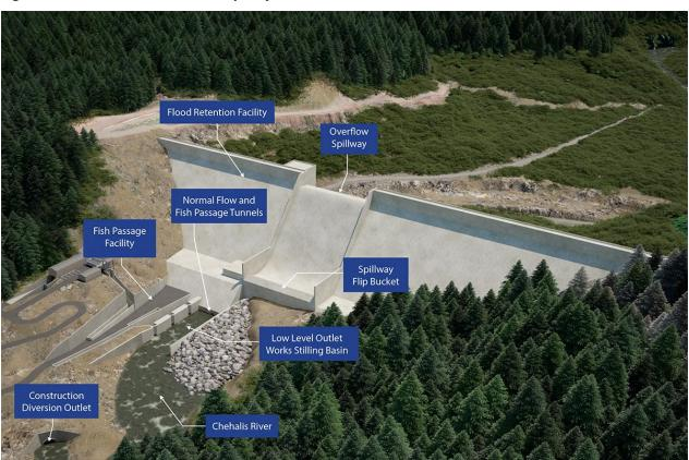
Figure 12-1. Flood Retention Facility Project.
