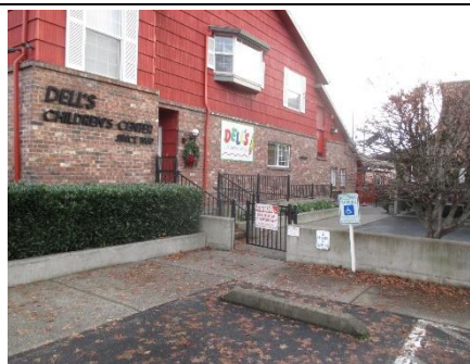
This floodwall can be seen on North Pearl Street in Centralia.
