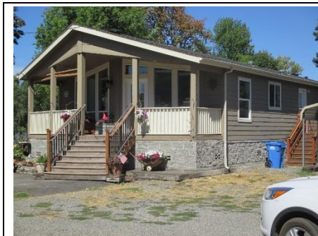
This house on the Chehalis River was elevated two feet above the base flood elevation.
