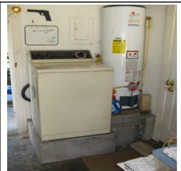
These appliances are elevated in a garage
